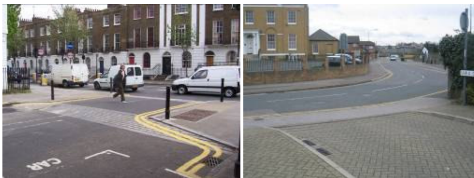
Pedestrian footway continues at one level, Islington (left) and Greenhithe (right)
