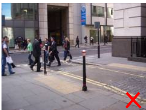
Incorrectly located crossover – not on the desire line for pedestrians – the crossover should be nearer the junction in this case with a steeper ramp for vehicles to come up onto it in order to use the side street.
