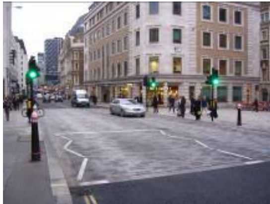
Carriageway graded to provide level crossing area on pelican crossings, Queen Street, City of London.
