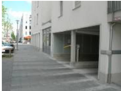
Image, Messestadt Riem, Munich Exit way (with control barrier) with kerbed footway to keep vehicles away from the wall in order to increase driver's line of sight to the right. Sight to the left is provided by the entry way. Note also the footway paving detail signalling to pedestrians the presence of a vehicle cross-over.
