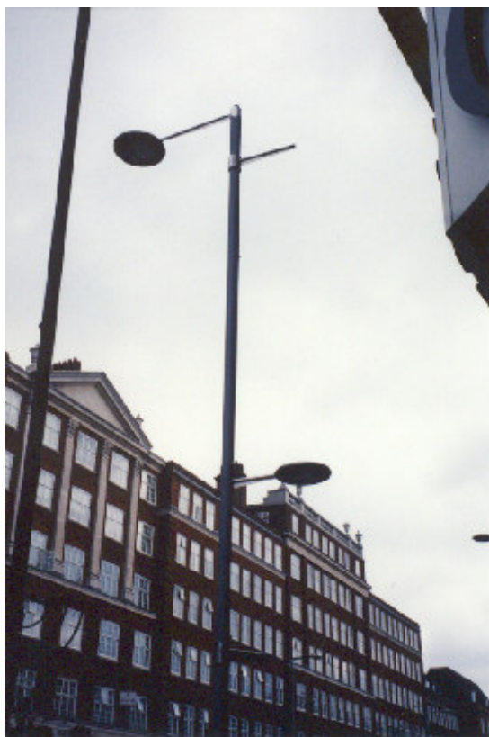
Piggyback lighting to illuminate footway as well as carriageway
