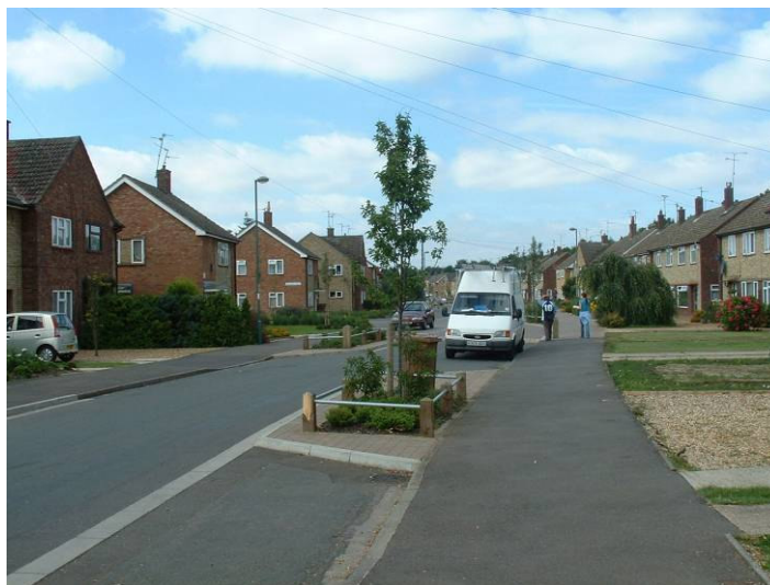
Kerb build out controls parking and locates street tree in highway space leaving footway clear, Peterborough
