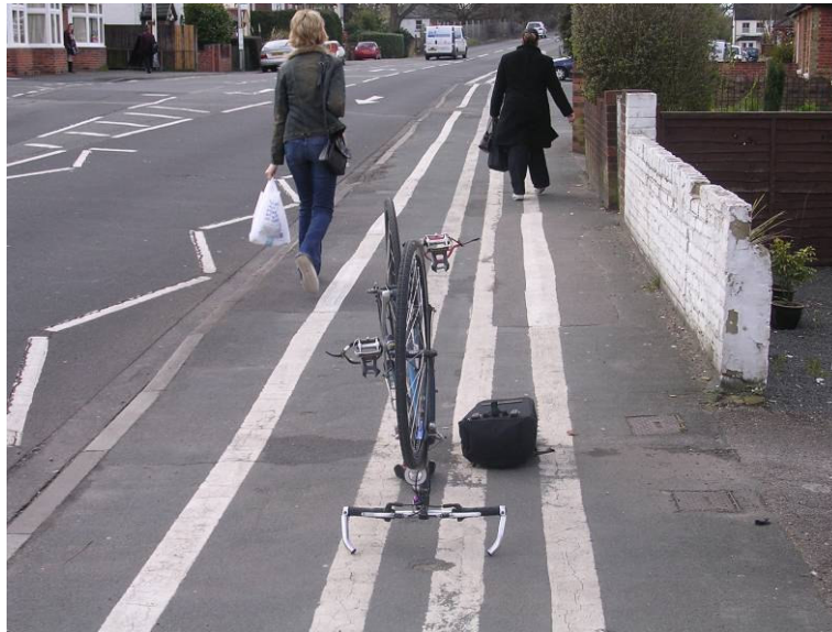
Poorly designed cycle facility: visually intrusive, confusing, unhelpful to cyclists
