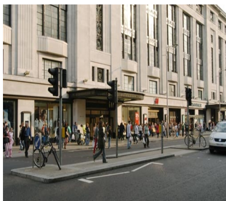
Staggered crossing with guardrailing removed
