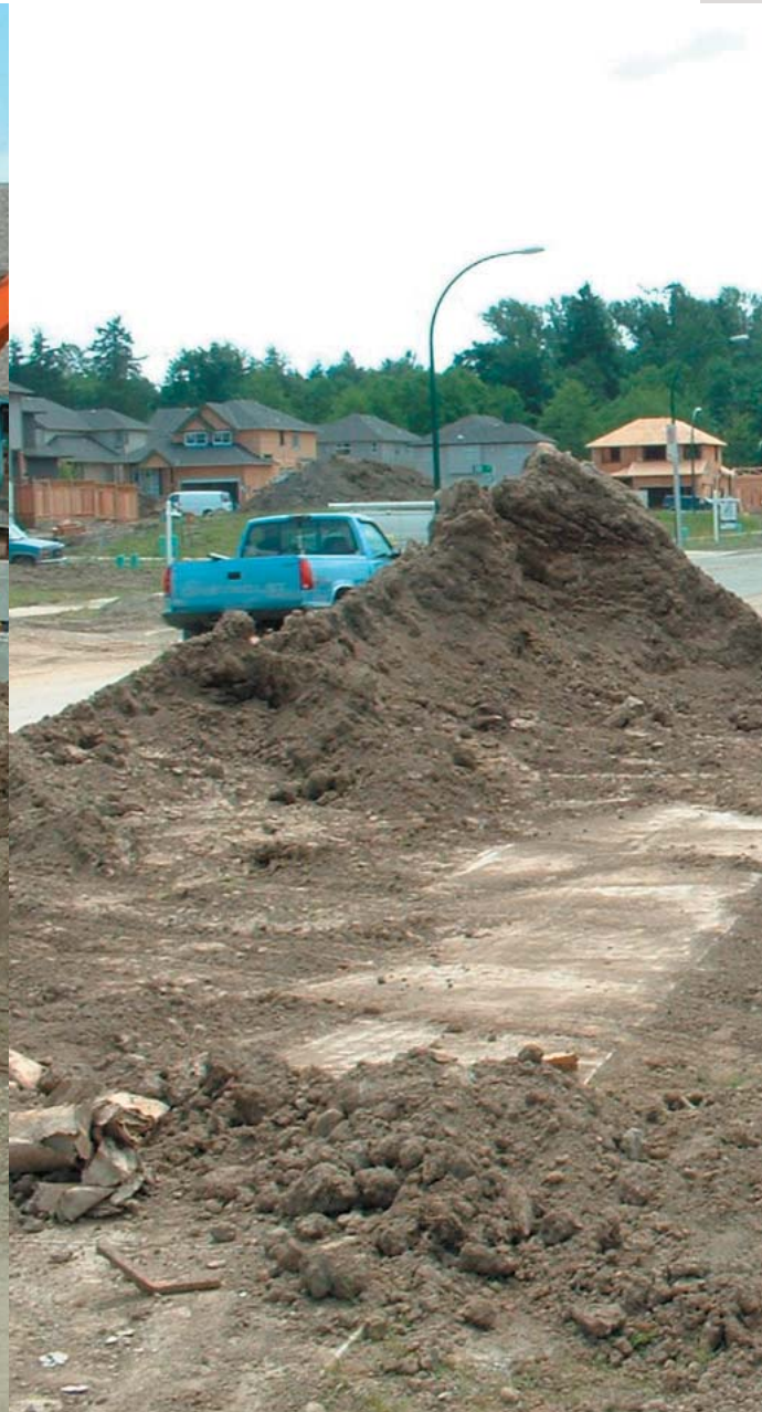
Left: infiltration devices in the form of crushed stone and clean out basins incorporated into front lawns. Right: topsoil to be replaced at double depth to absorb water.
