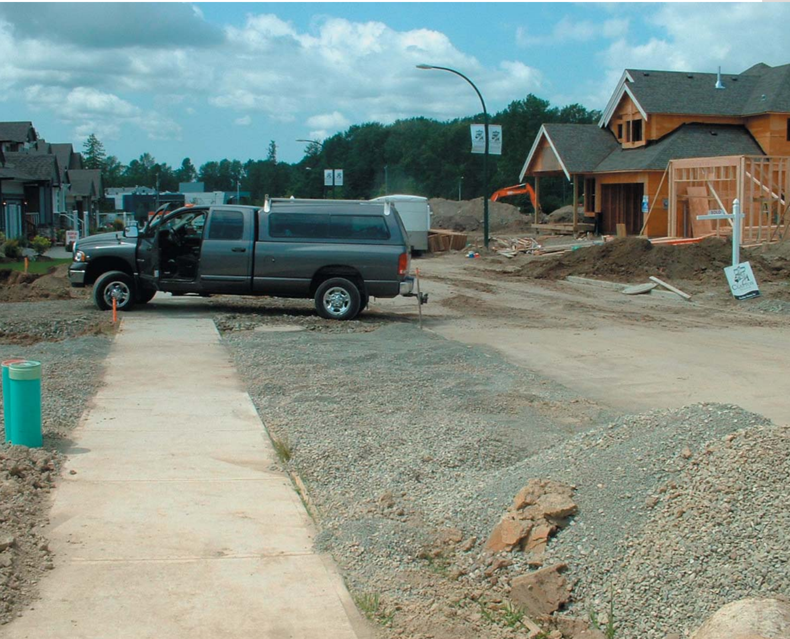
East Clayton back lane providing rear vehicle access to residences.
