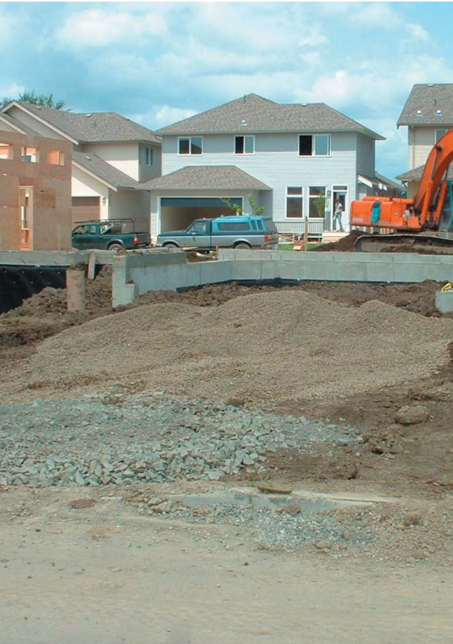
Left: infiltration devices in the form of crushed stone and clean out basins incorporated into front lawns. Right: topsoil to be replaced at double depth to absorb water.
