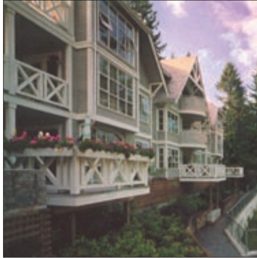
Photo source: Aplin and Martin Consultants Ltd.
