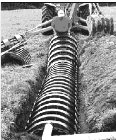
Figure 3-1 - The High Capacity Chamber units are 34" wide, 75" long, and 16" tall and designed to fit into a three-foot wide trench as a direct replacement for stone and pipe. (See figure 2) The system can be installed by just two people, one on a backhoe and the other installing the polytuff (TM) units.
