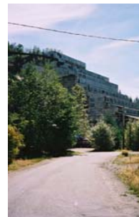
Storm Drains are non-existent Photo: J. Lommerse
